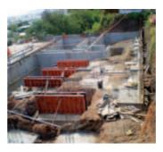
Three standard lightweight panels measuring 120, 90 and 60 cm available in two heights of 210 and 180 cm (multiple 30 cm modules)
