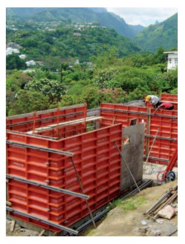
The special configuration of the edge section in the **steel mini** system interacts with the clamp to ensure smooth coupling and locking with just the simple tap of a hammer.
