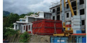
The panels have been designed around a 30 cm module and can be positioned both vertically and horizontally to meet the geometrical requirements of the form-worked wall in the best manner possible.
