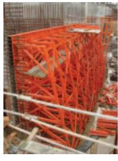
We set ourselves the task of designing and testing a simple, fast coupling system which would ensure that panels were perfectly coplanar (no offset), well-locked (no loss of grout) and accurately aligned (no additional stiffening for handling over large surface areas)
