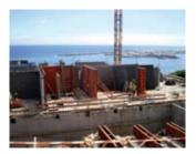
panels weigh only 35 kg/m² and can easily be handled without a crane;
