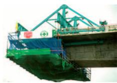
The **alpi sea** Balance Cantilever system is used for the **cantilevering method of construction**, This kind of equipment can be used for placing prefabricated segments (Length of segments are approx. 3-5 m) or for cast in situ concrete.
