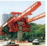
In fact, Launching Gantries are most often used for placing prefab segments, match-cast and stressed together or in complete units, spanning from pier to pier.
