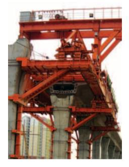
alpi sea's Launching Gantry (LG) method of construction has been developed for multi-span bridges over difficult terrains or water where scaffolding is expensive or not feasible at all.
