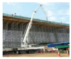
factories, power plants, water towers, recycling plants, refineries, incinerators, large scale performance stages etc. for both Falsework and access such as in viaduct construction, where complete towers sets can be moved horizontally using special trolleys and rails, then simply crane lifted to the next location, saving time & labor costs.
