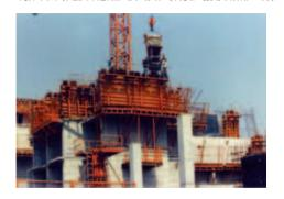
Climbing systems brackets provide the supporting structure for Formwork for successive off-ground casting operations. With weightbearing rests on the attachment anchored to the cast, while a safety
