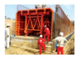
as arches or any type of tunnel work **alpi sea**'s tunnel Formwork Systems operate manually or are self propelled which is particularly cost-effective since 80% of the carriage consist of **alpi sea** standard products such as panel & scaffolding systems.
