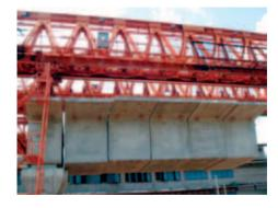
For both construction methods "span by span" and/or "cantilever", the framework consists of two (2) lattice trusses with a triangular section, the ends of which are connected via horizontal bracings.
