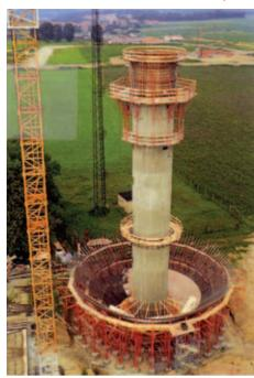
The platforms rest directly on a wall recess, on a special support device previously fixed to the wall.
