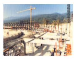
This 30,000 seat outdoor stadium has been built for the S.E.A Olympic games with alpi sea's steel Formwork and Falsework Systems. The challenge of this project was to provide a combination of equipment made of alpi sea standard products such
