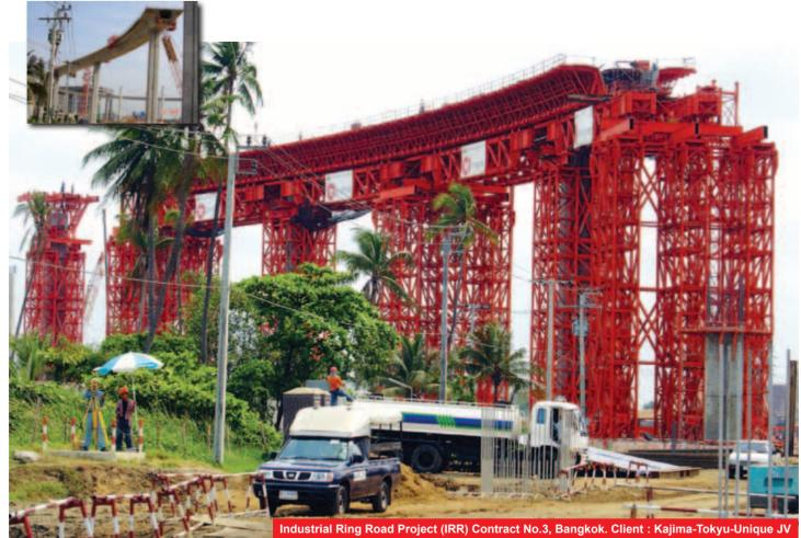
A transportation system (Rebar trolley) for prefabricated reinforcement cages, or a portal crane system can be integrated within the entire system.
