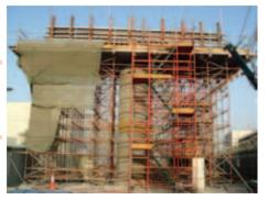
lower cap, which is welded to the vertical at 0.5 m intervals, with a sliding upper cap. The forged blade ends of the horizontals are located in the lower cap. The upper cap is moved down and rotated by hammer blows to give a positive and rigid connection.
