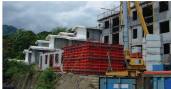
The panels have been designed around a 30 cm module and can be positioned both vertically and horizontally to meet the
