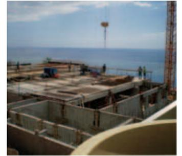
Using a limited number of components, formwork can be set up for any kind of structure from the simplest to the most complex, from foundations and bases to intricate wall systems. Using cranes for large surface areas or mounting panels individually by hand.
